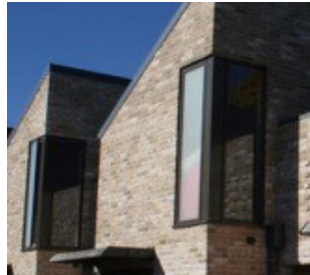
Fig. 68 - Corner windows and terraces are positive features
