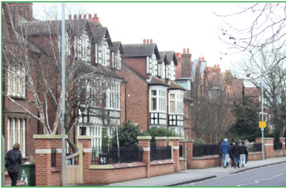
Row of detached villas
