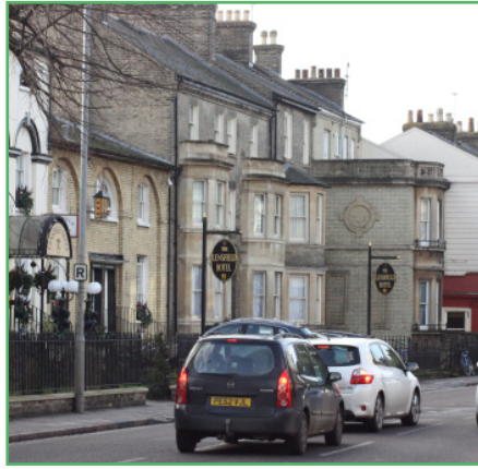
Later additions to No. 65
